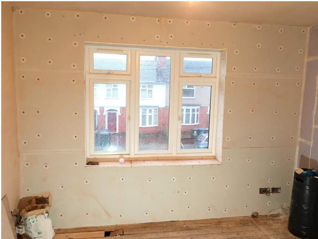
Plasterboard / Fixing – Fig 6
