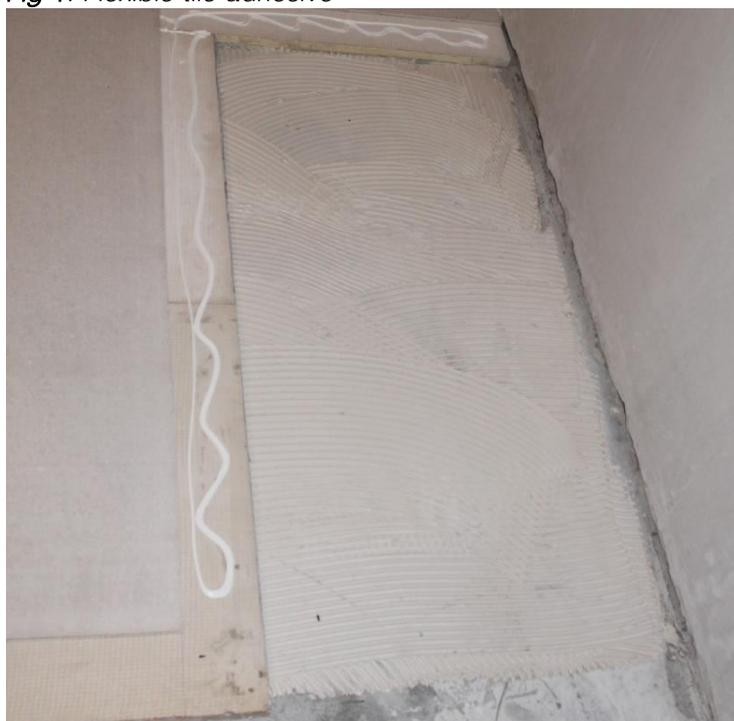
*Fig 2 E-Therm Slim ship lapped on flexible tile adhesive*
